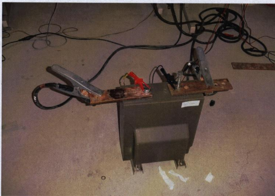
Figure 2: EUT under measurement of resistance
