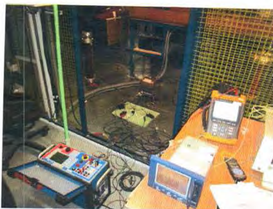
Figure 4: Measurement of DC resistance of windings
